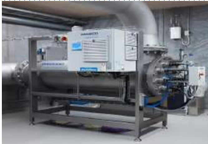
Ultraviolet water disinfection system
