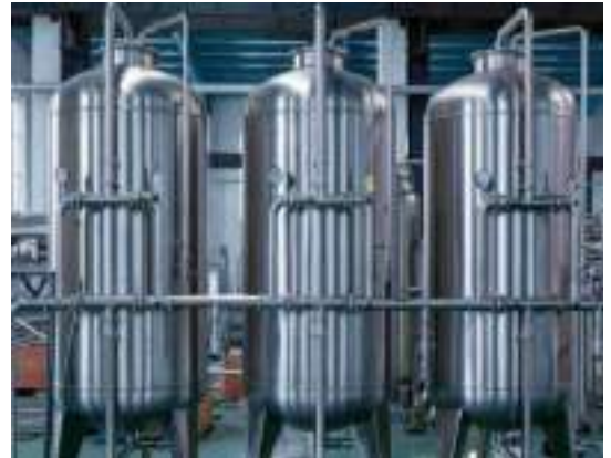
Pic.1 Water filter system
